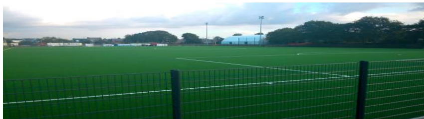
FIGURE 2 : TERRAIN DE FOOTBALL SYNTHETIQUE A LOCUNEL
